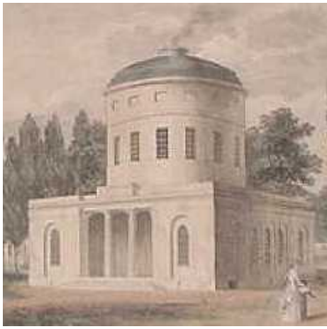
Center Square Pump House
