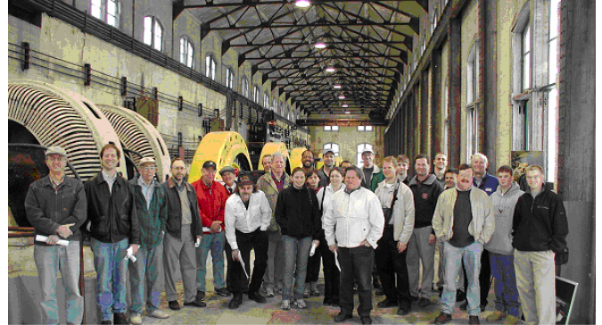
Our tour group inside the generating station
